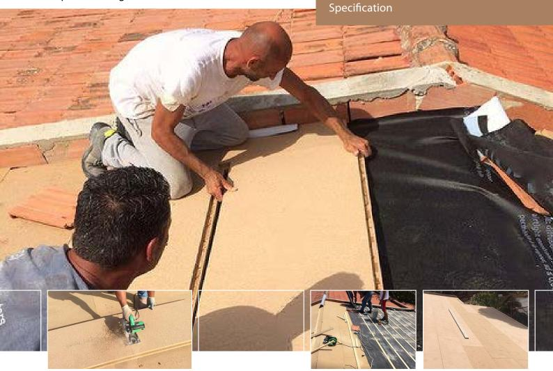
THERMAL INSULATION FOR NEW ROOFS OR RENOVATIONS
