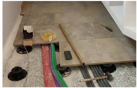
Laying laser-level supports fixed to the base and head with screws and plugs on BetonWood
